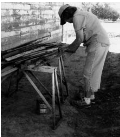
Above, work inside the Toltec Schoolhouse. Below, Kethleen Krider removing nails from lath. Photos by Donna Bengé
