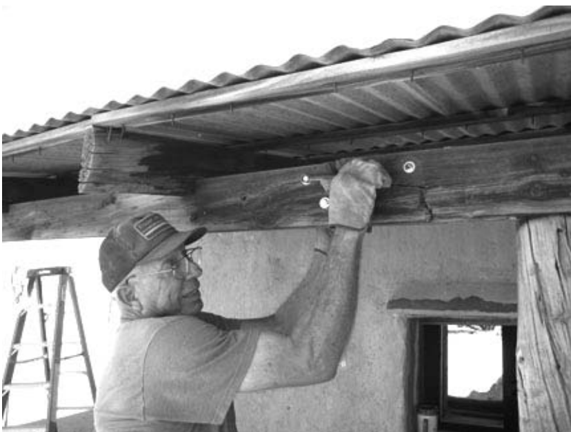
Dick Myers repairs a porch beam at the stage stop.
