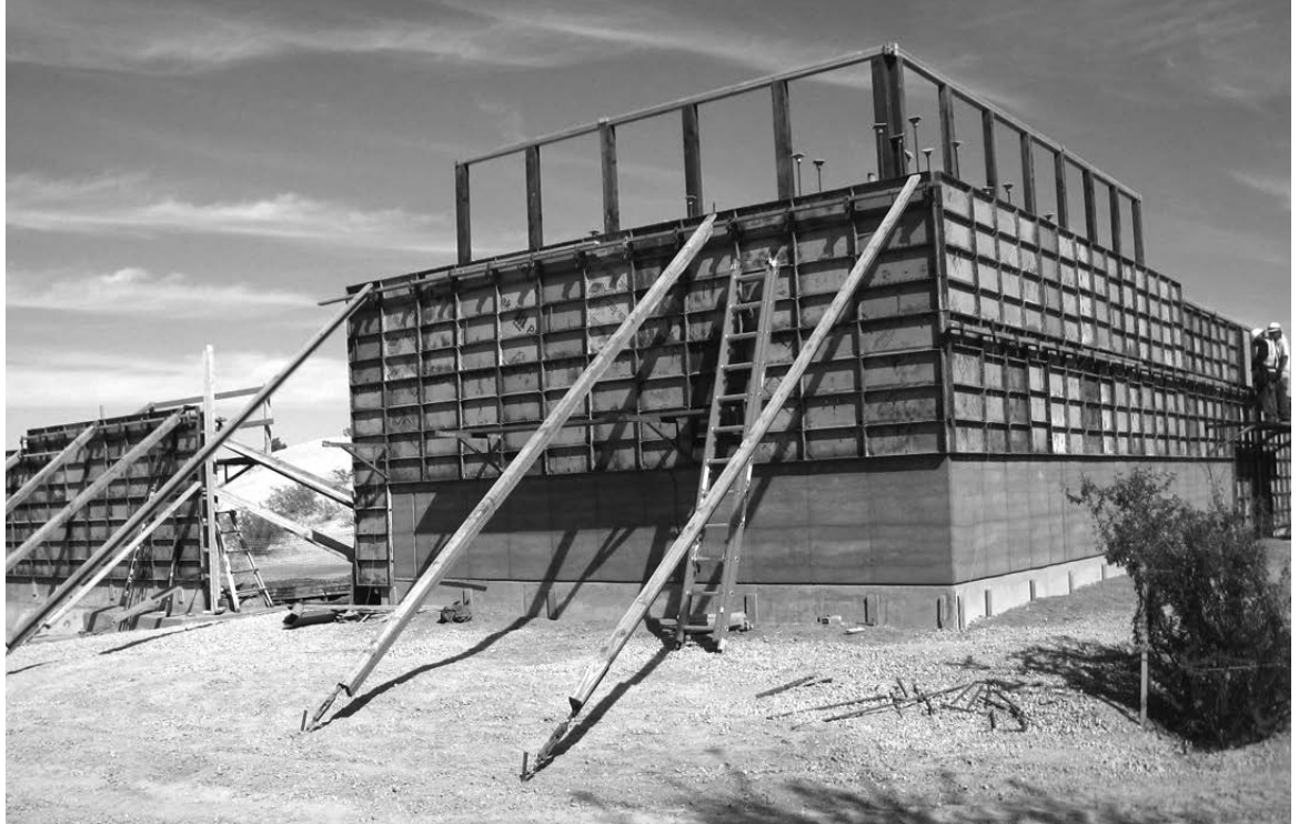
Construction under way for the visitors' center at Mesa Grande mound.
