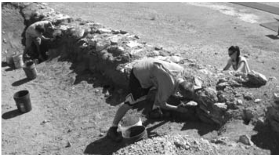
Stabilizing the wall of "Miller's Room"
