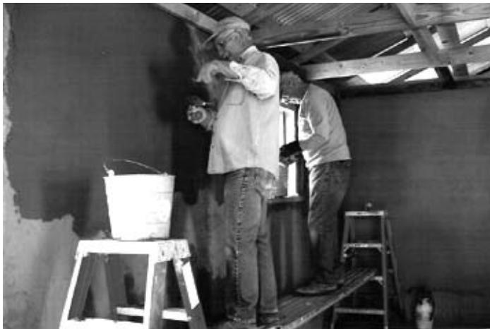
Jim Britton and Dick Myers adding fine mud plaster at Verdugo
